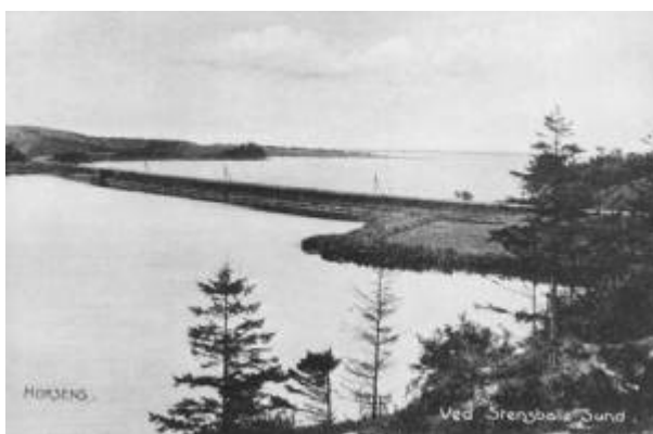
Jernbanebroen over Stensballe Sund 1904
